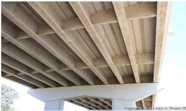
Intermediate and End Diaphragms between Girders
