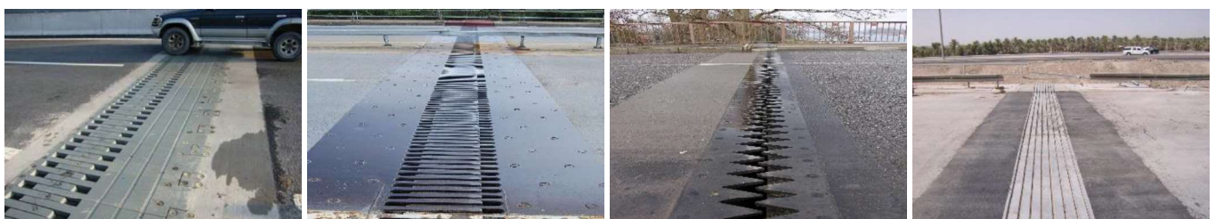
Figure 1.10: Typical Expansion Joints of Bridges
