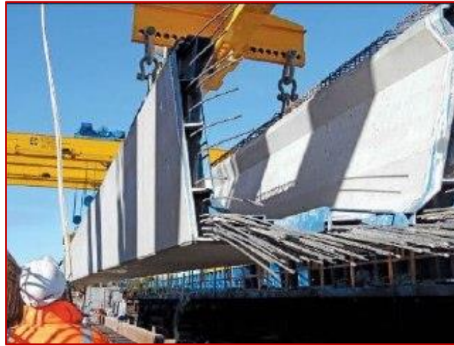
Fig (19) pre-stressed concrete beam
