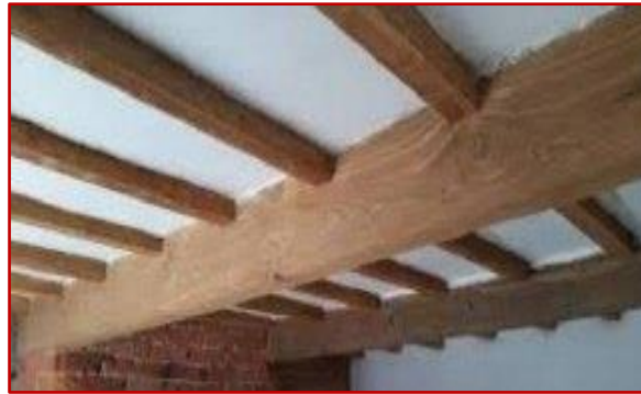
Fig (7) timber beams
