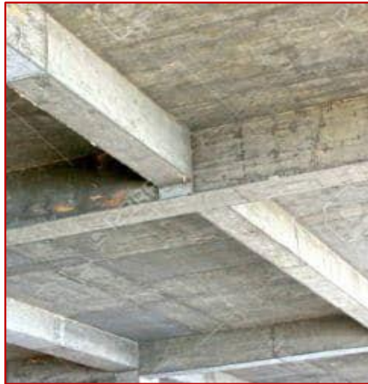
Fig (17) cast in-situ concrete beam
