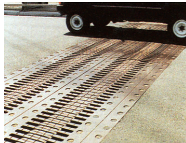
Fig. 12–15 An expansion joint on a bridge.
