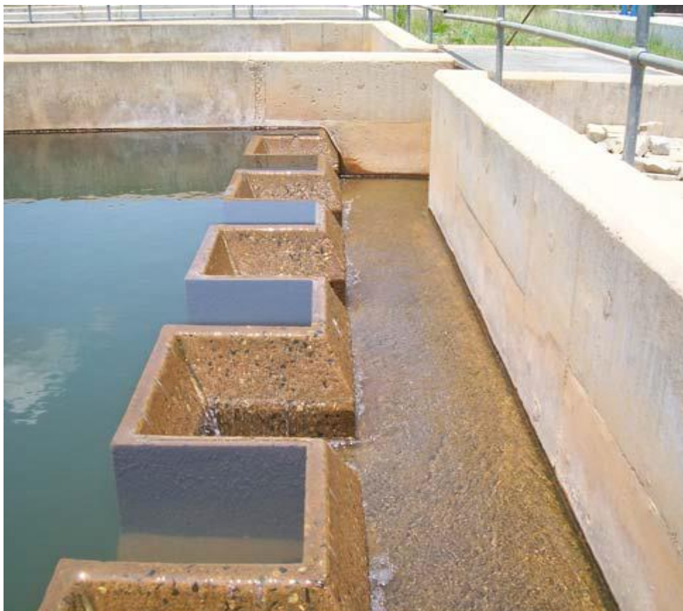
Fig. (13) Finger weirs
