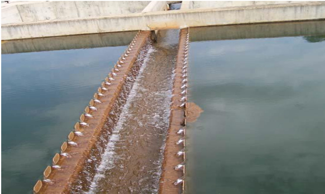
Fig (12) typical effluent structure
