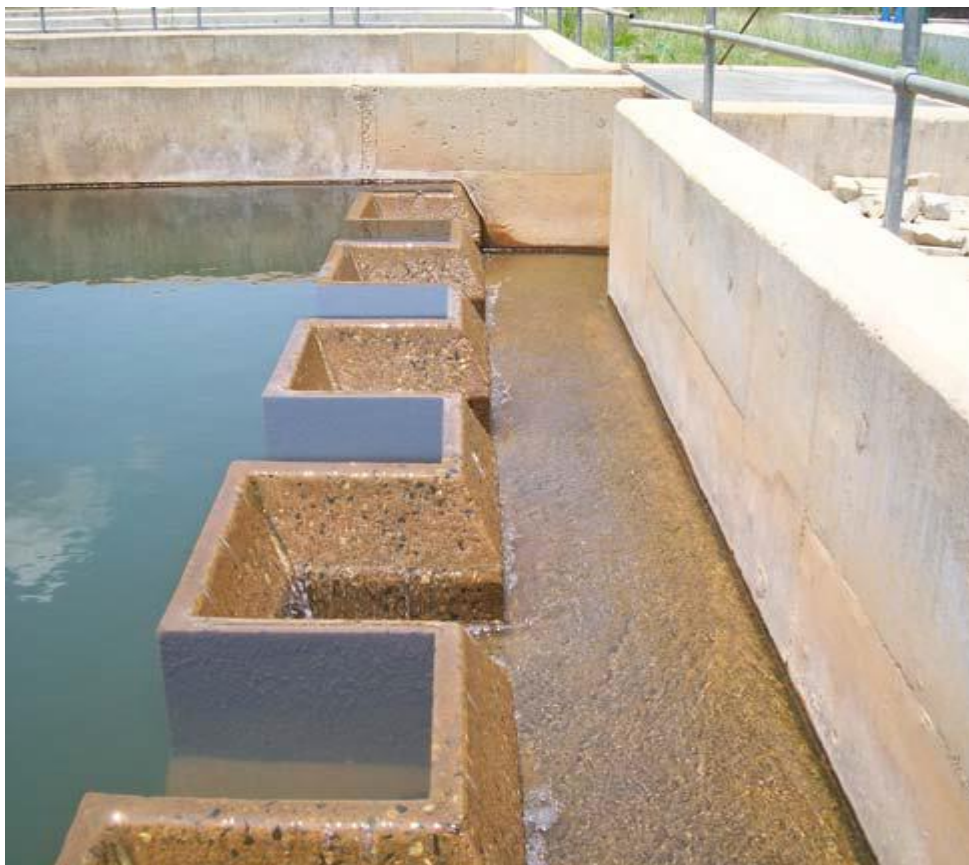
Fig. (13) Finger weirs
