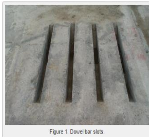
Figure 1. Dowel bar slots.
