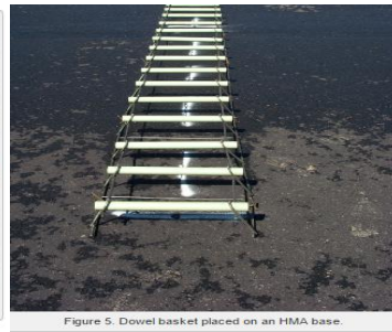
Figure 5. Dowel basket placed on an HMA base.
