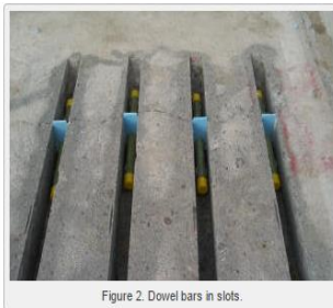
Figure 2. Dowel bars in slots.
