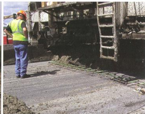
Figure 5. Dowel basket placed on an HMA base.
