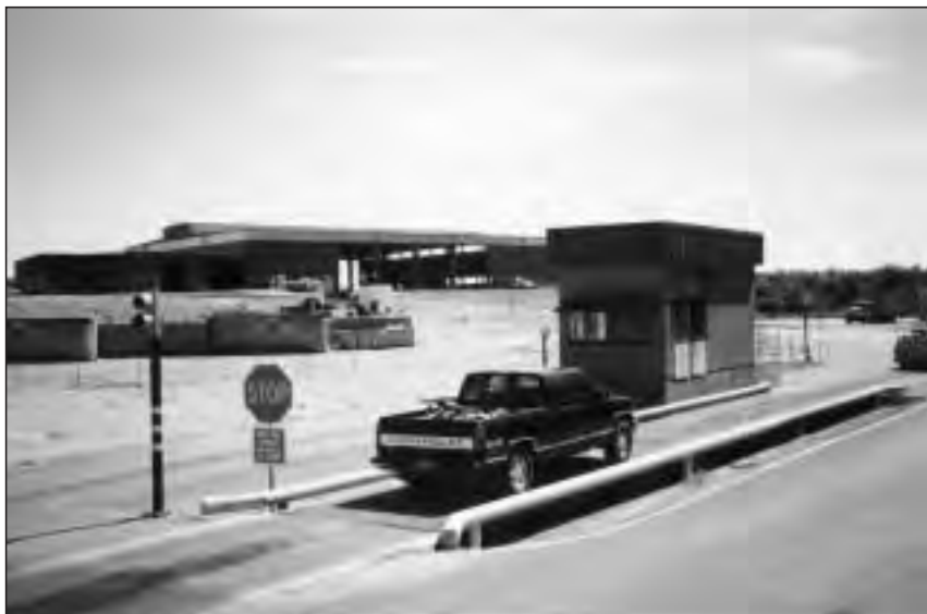
A transfer station scale house.
