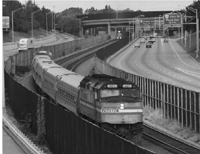
Figure 14.3 CSX Railroad in the median of I-195, Richmond, Virginia
