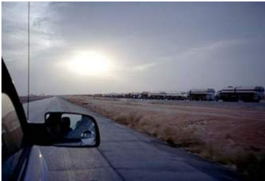
Figure: Typical Two-Lane, Two-Way Highway in a Rural Environment.
