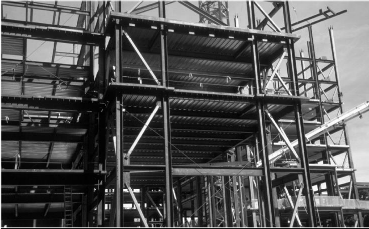
Figure show columns, beams & bracing
