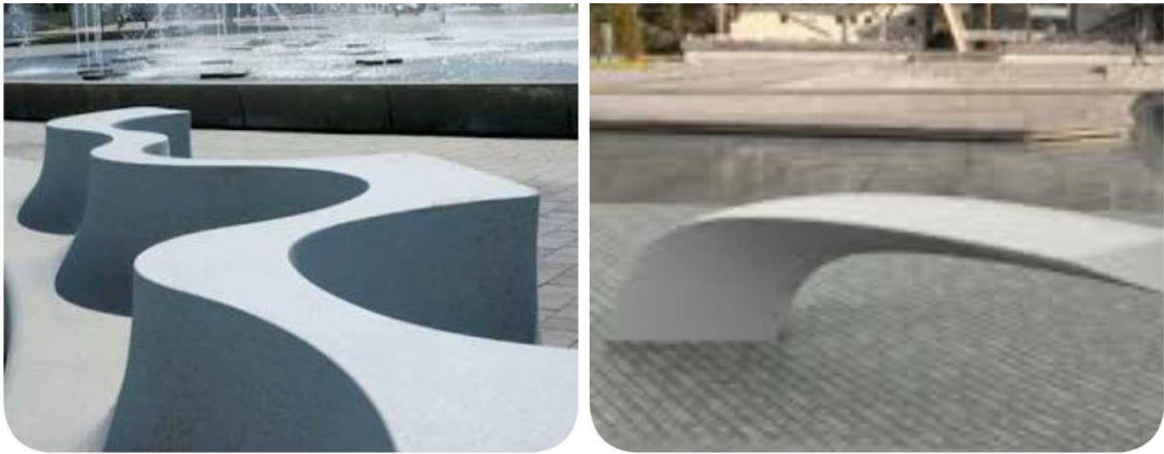
Seating Benches Constructed Using SCC
