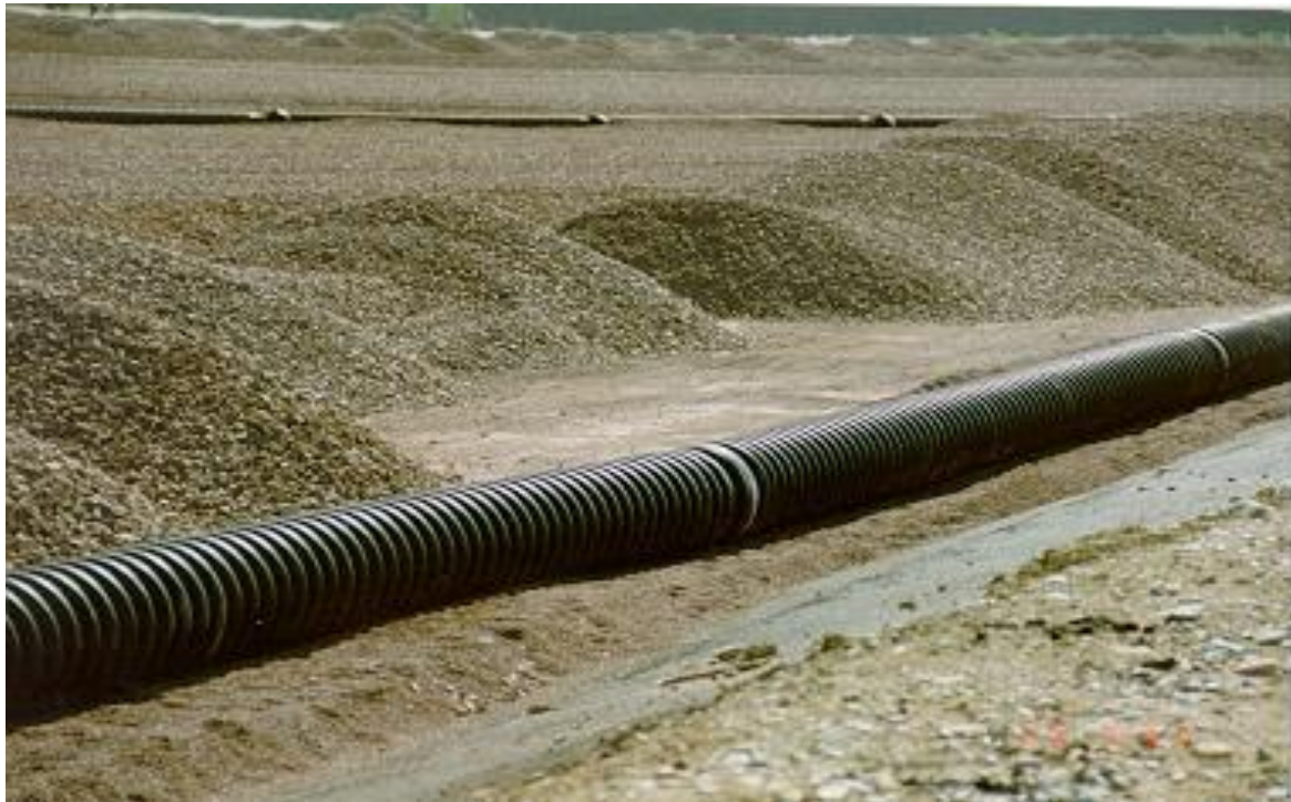
Fig. 5 Leachate (wastewater) collection system
