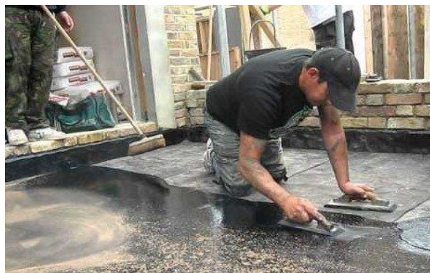
Fig.(13): Asphalt Flooring
