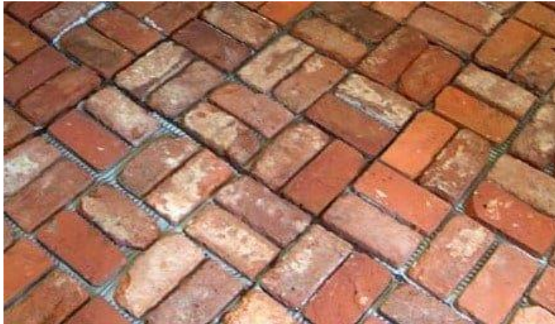
Fig.(2): Brick Flooring in Buildings
