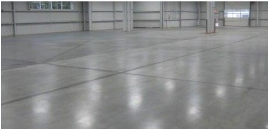
Fig.(1): Cement Concrete Flooring
