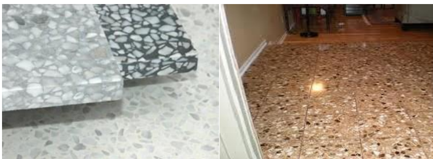
Fig(5): Terrazzo flooring
