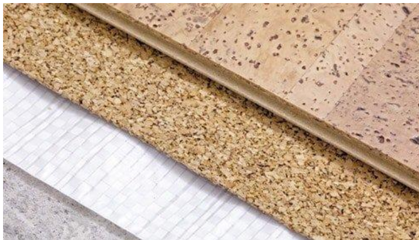
Fig.(11): Cork Flooring in Buildings
