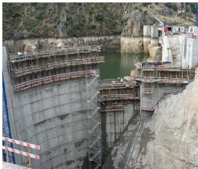
Fig 1: Construction of Dam using Low Heat Cement.
