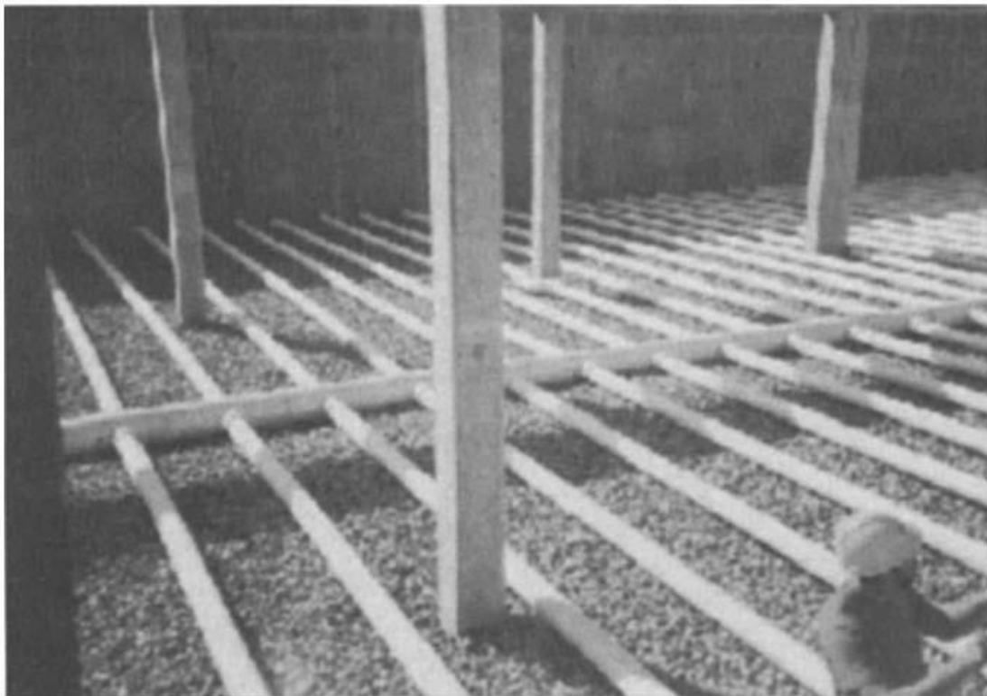
Figure (7.8): Underdrain installation
