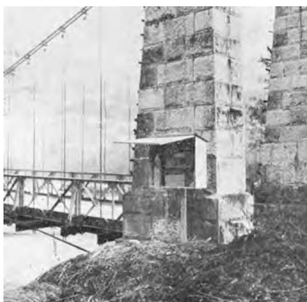
Fig. 4.5 Bubble Gauge Installation— Telemip (Courtesy: Neyrtec, Grenoble, France)
