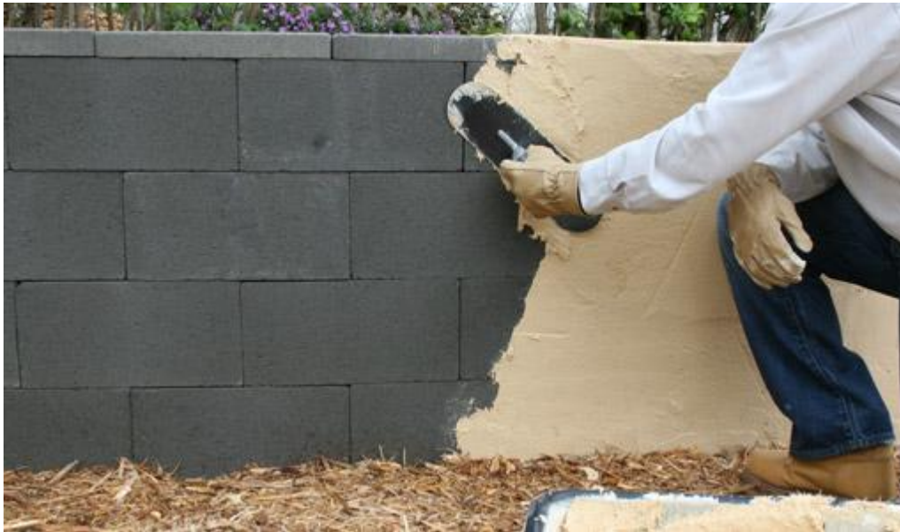
Figure (3): Applying surface-bonding cement to a dry-stacked, concrete block wall
