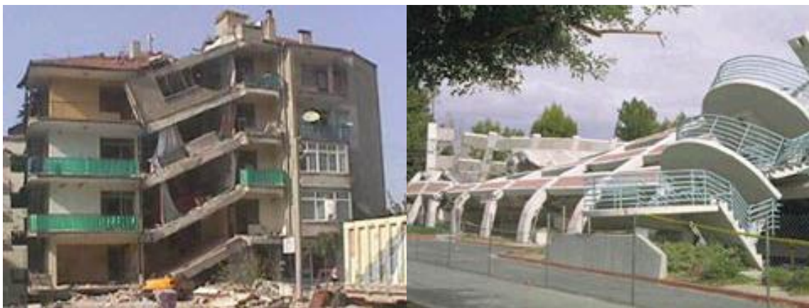
Figure 1: Collapsed structures destroyed by the shallow 1999 Izmit, Turkey (left), and 1994 Northridge, California (right).
