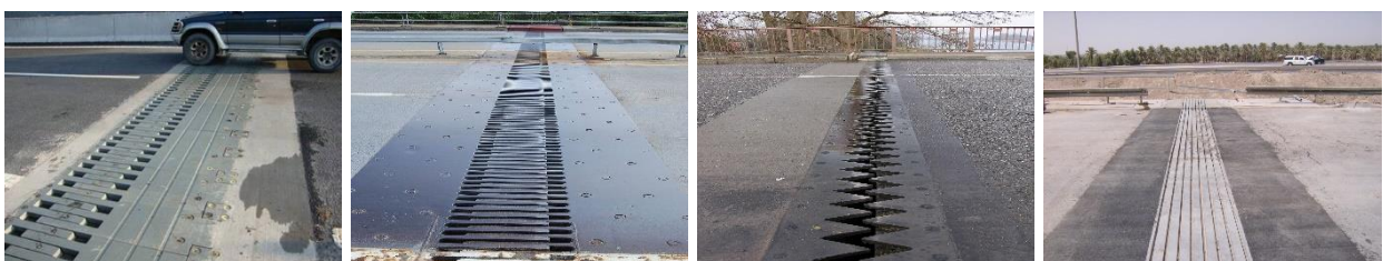
Typical Expansion Joints of Bridges
