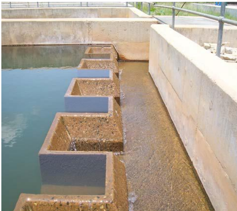
Fig. (13) Finger weirs
