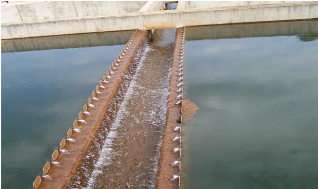
Fig (12) typical effluent structure
