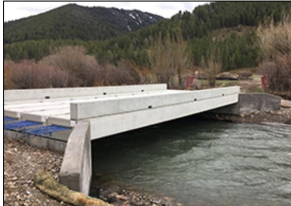
Figure (7) Simply Supported Slab Bridge
