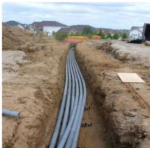
Fig. 5 –4 Direct Laying of underground cables
