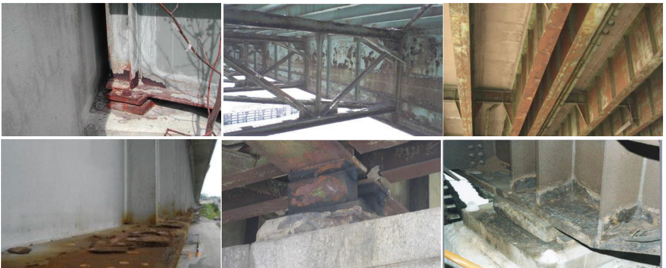
Figure 2.1: Corrosion of Structural Steel in Bridges
