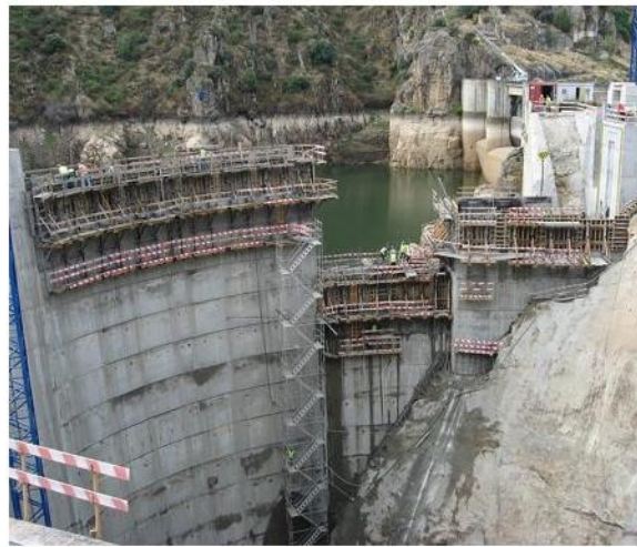
Fig 1: Construction of Dam using Low Heat Cement.
