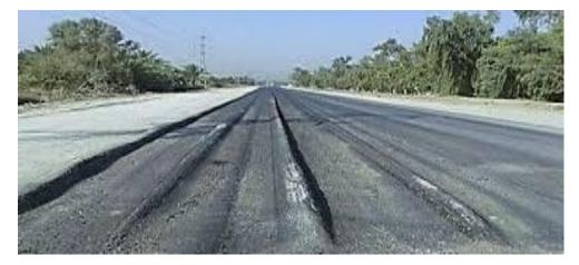
$\rightarrow$  Harder grade  $\rightarrow$  Low temperature cracking
