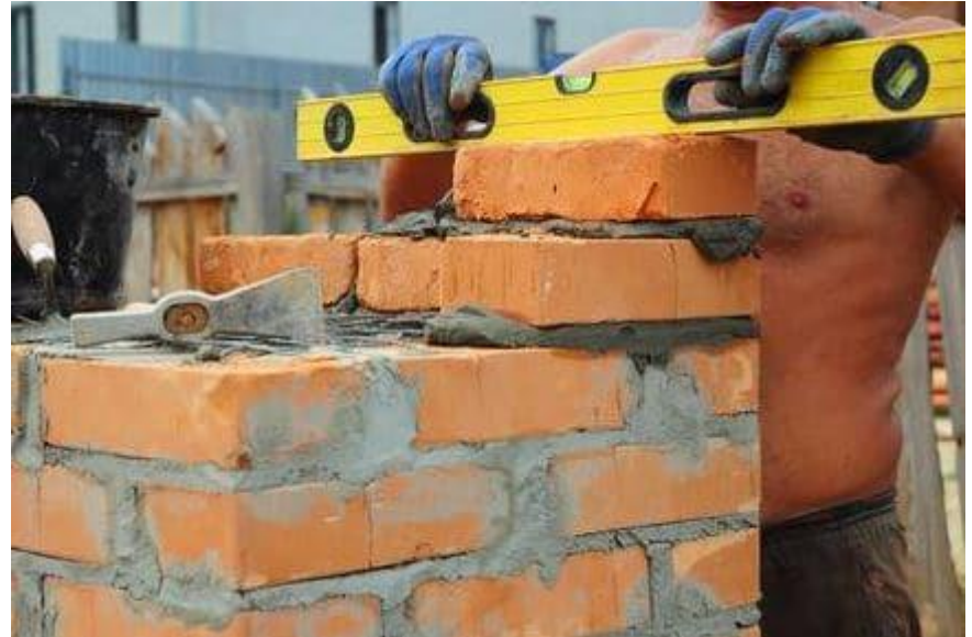
Fig. 8: Checking level of brick masonry
