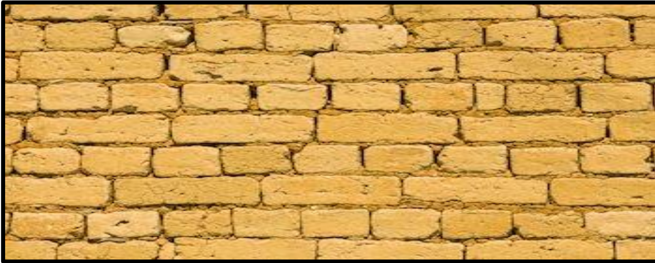
Fig. 1: Brick work in mud
