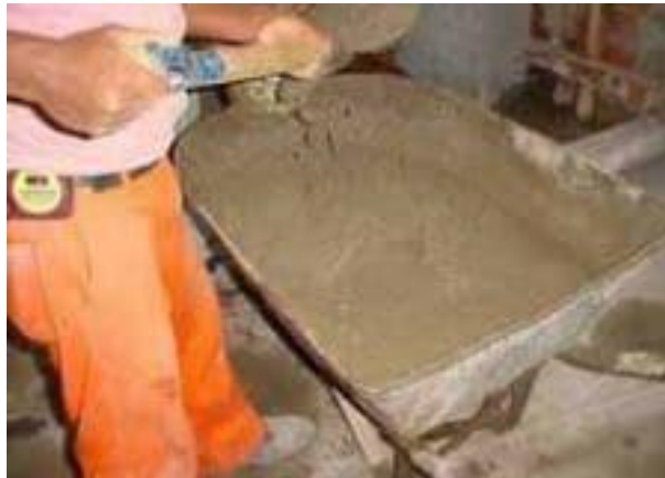
Fig. 5: Mortar Preparation
