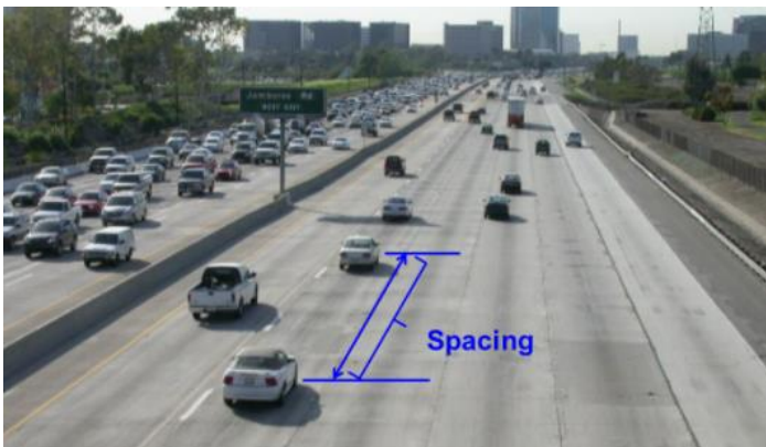
Uninterrupted facilities roadways
