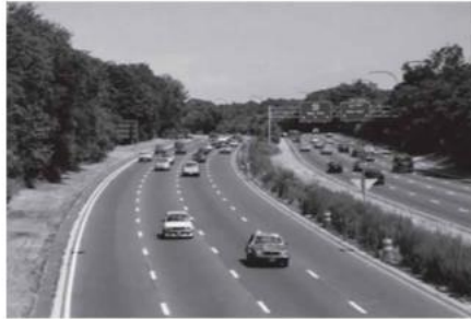
(a) A Typical 8-Lane Freeway
