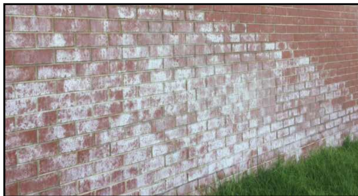
Fig.7 Efflorescence on brickwork
