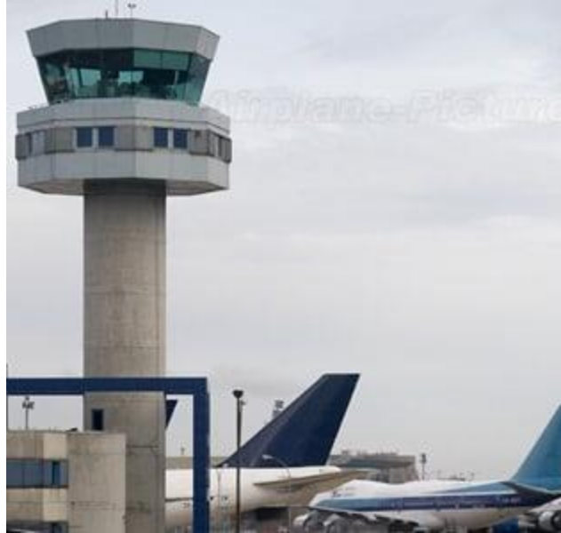
. Fig. No.6 :control tower
