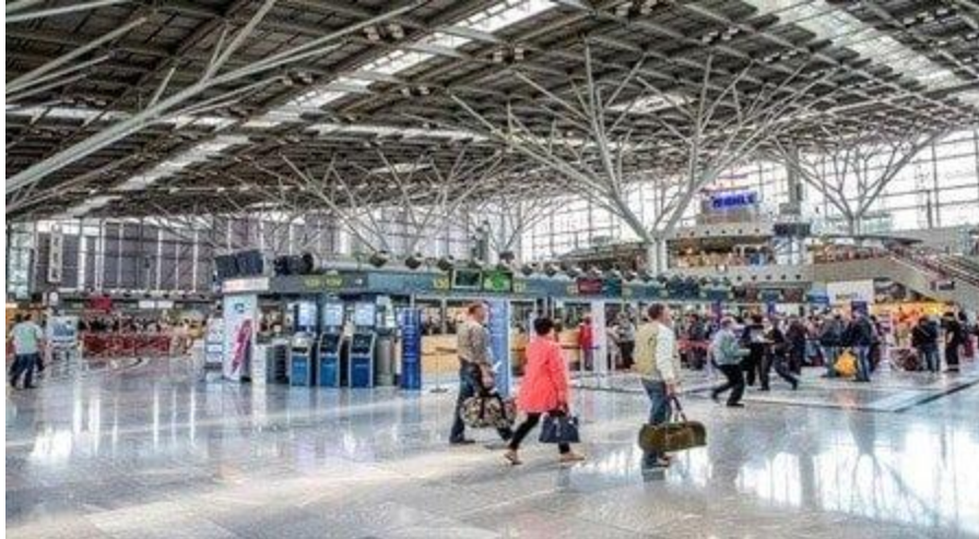
Fig. No.5: Terminal Building
