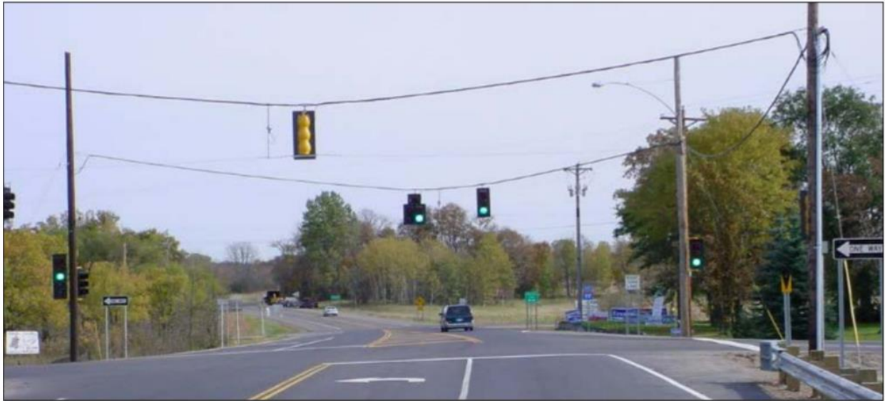
Figure 30: A Typical Span-Wire Signal Installation.
