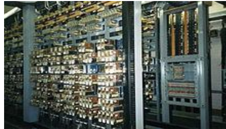
Part of a relay interlocking using miniature plug-in relays
