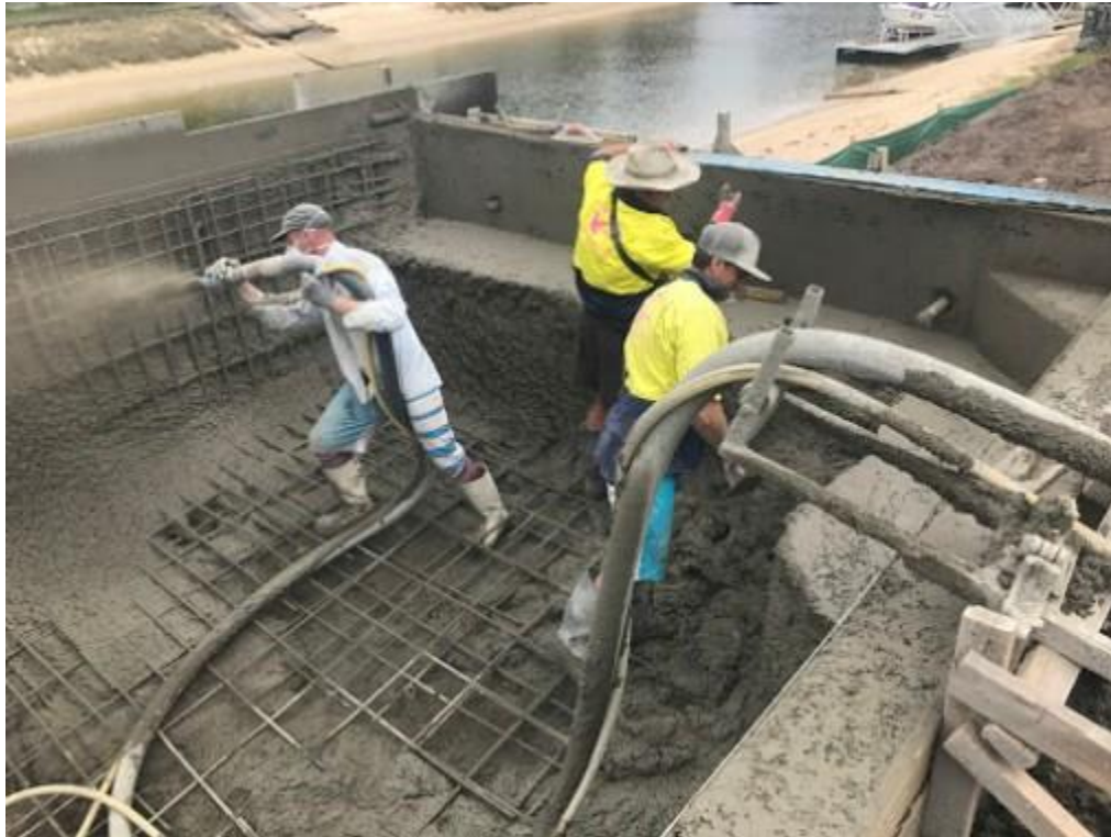
Concreting in Swimming Pool Construction
