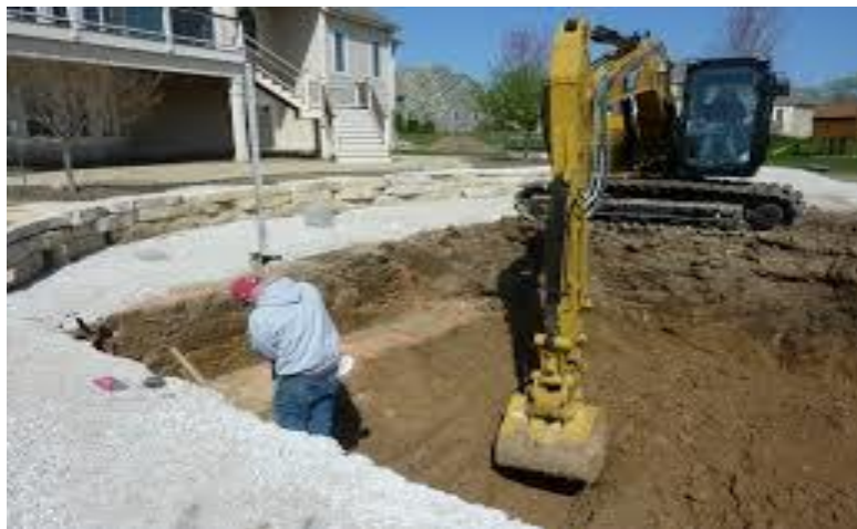
Excavation for Swimming Pool Construction
