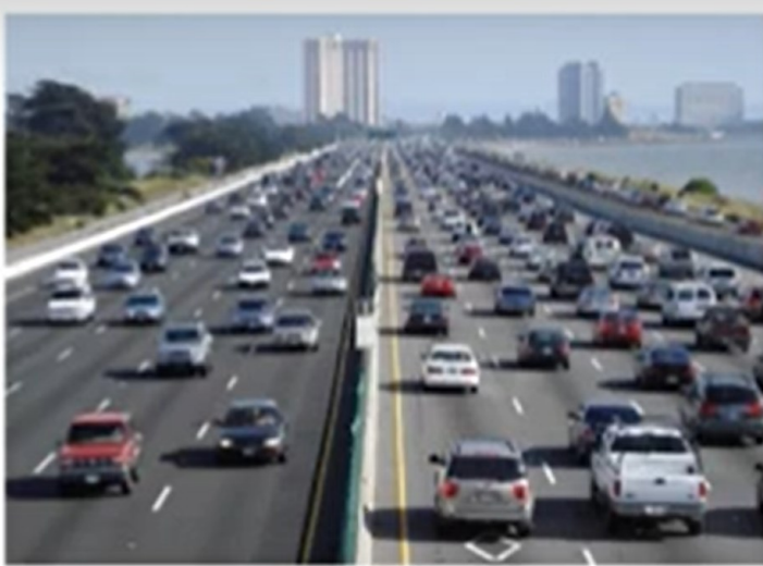
(a) A Typical 10-Lane Freeway
