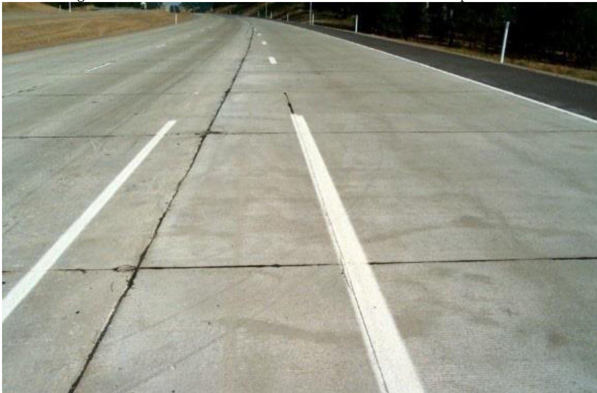
Fig.7: Jointed Reinforced Concrete Pavement
