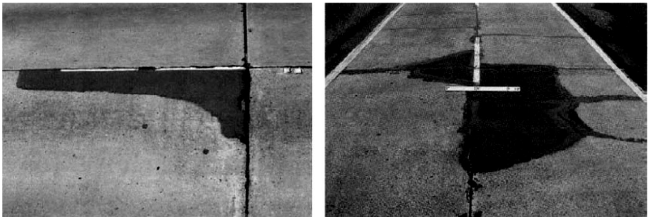
Figure (19-C) Patches in rigid pavements
