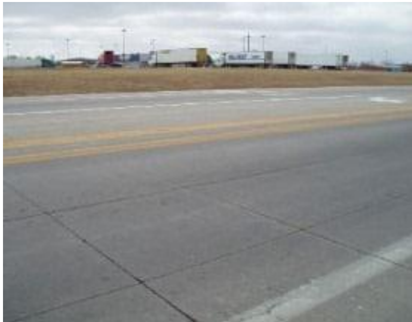
Fig.2: Jointed Unreinforced Concrete Pavement
