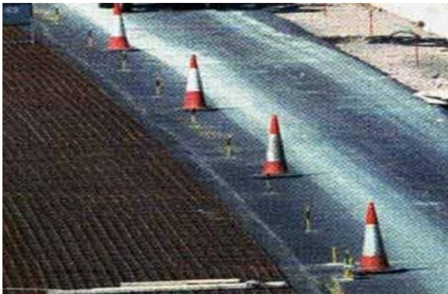
Fig.10: Continuous Reinforced Concrete Pavement with Successive Whisper Concrete Resurfacing
