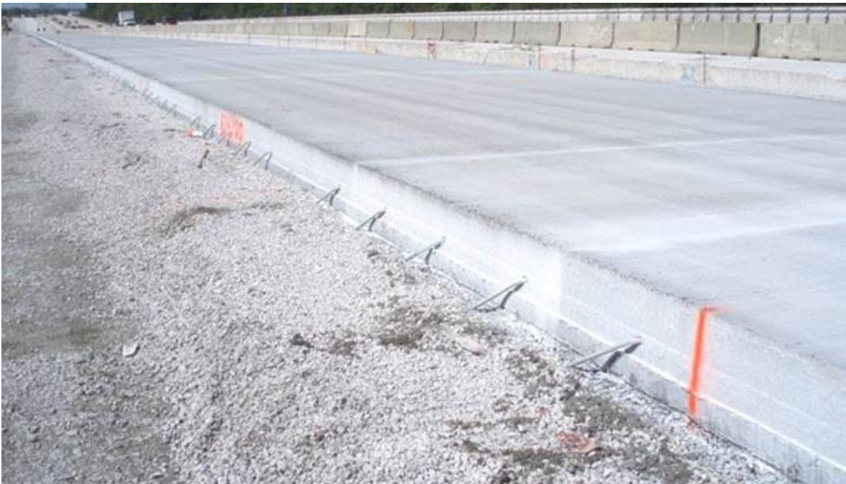
Fig.1: Concrete Pavement Constructio
