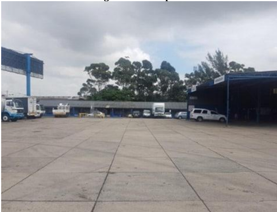
Fig.6: Industrial Yard Constructed using Jointed Unreinforced Concrete Pavement
