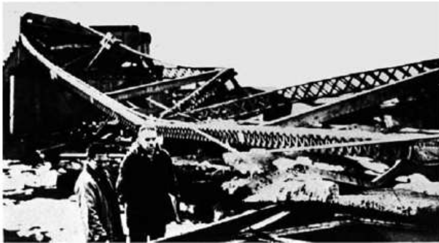
Figure 2: On December 15, 1967, the silver Bridge connecting Ohio and West Virginia over the Ohio River collapsed, and 46 people lost their lives. The case of the collapse was stress-corrosion.
