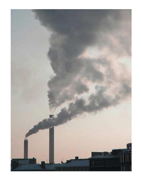
• Gases leaving the tops of stacks rise higher than the stack top when they are either of lower density than the surrounding air (buoyancy rise) or ejected at a velocity high enough to give the exit gases upward kinetic energy (momentum rise).
